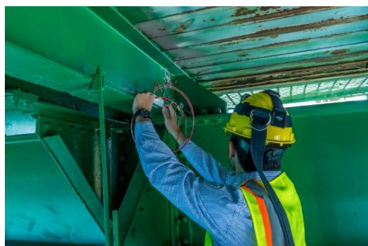
© Michigan State University Self-powered piezoelectric-floating-gate sensors being attached to a bridge to monitor and store data about the structure.
