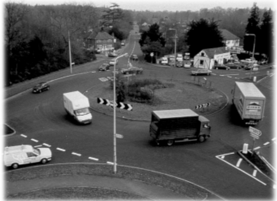
Roundabouts: An Informational Guide provides background information and discusses the safety and operational benefits of roundabouts.
