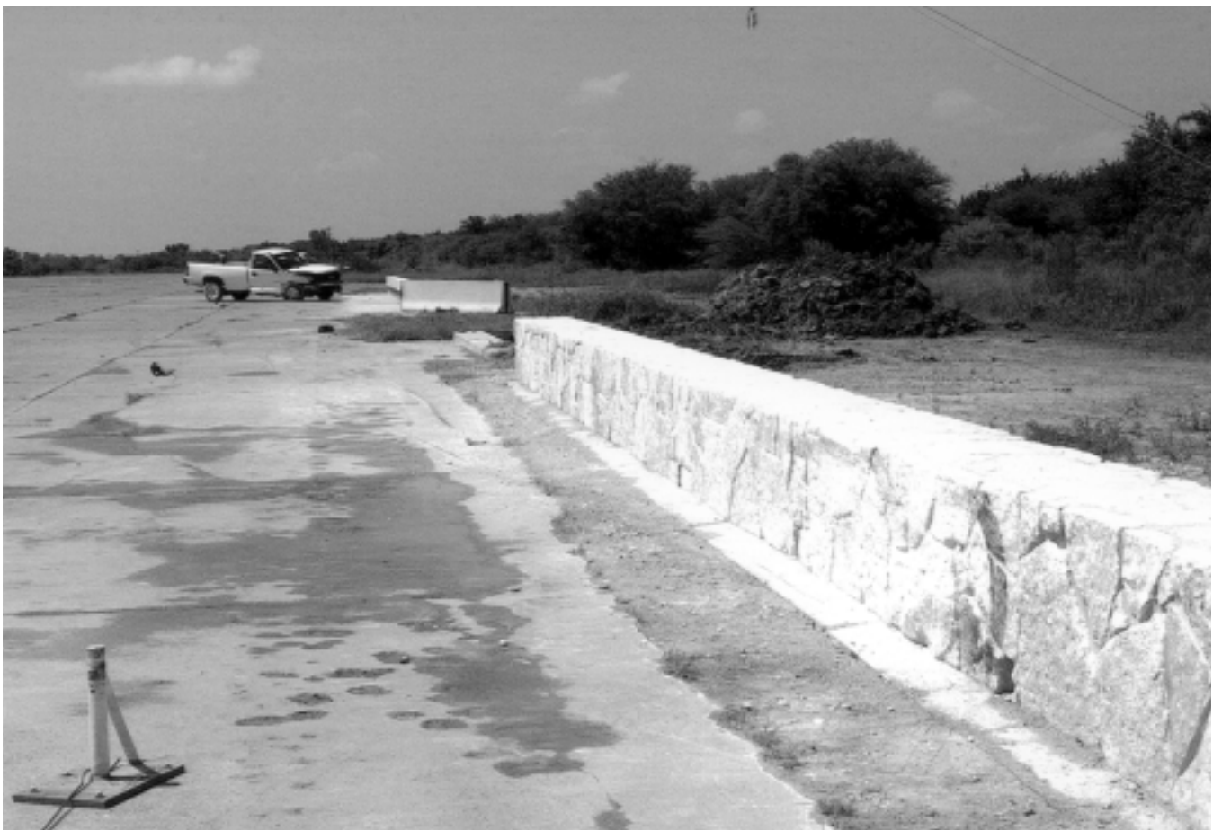
Rough stone masonry guardrail after the crash test.
