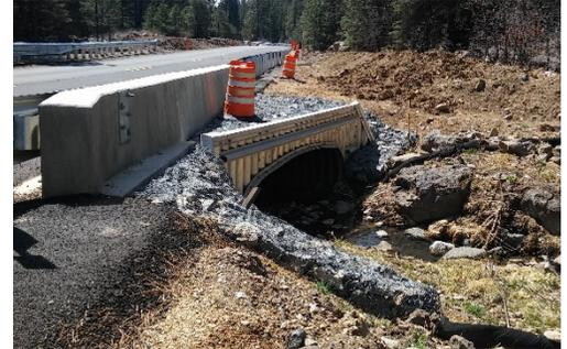
A bottomless culvert was installed under NM-434 to connect Big Blue Creek, a tributary to Coyote Creek, with NM-434.
