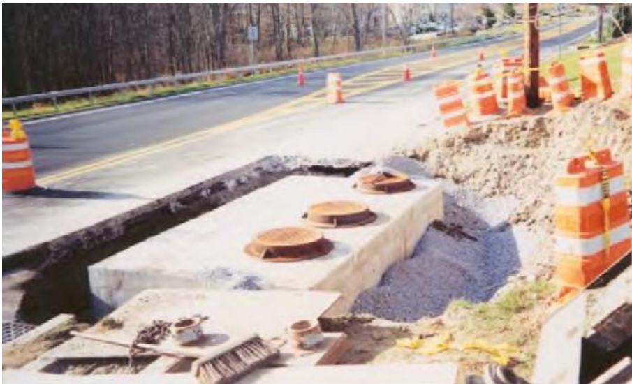
Photo of a vault in New York State. Maintenance requires lane closure. (Photo by NYSDOT.)
