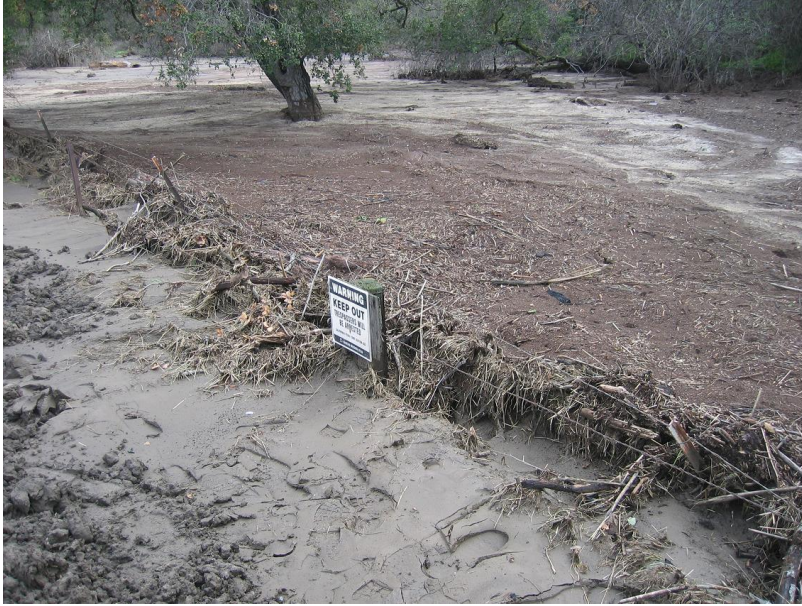
Photo depicting mudflow at SR-74 emergency slope and culvert repair project, Orange County, 12-2010. (Photo by Caltrans D12 Maintenance and Engineering Department.)
