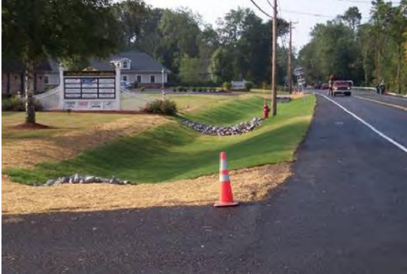
Photo of Swale in New York State. The design was limited by right-of-way and for safety. Some pollutant sources originate from outside of the DOT right-of-way. (Photo by NYSDOT.)
