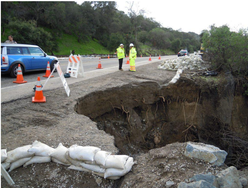
Photo showing erosion and slope failure at SR-74 emergency slope and culvert repair project, Orange County 01-27-09, Federally endangered arroyo toad habitat. (Photo by Sally Brown, USFWS.)
