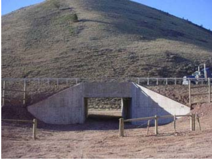
Photo of a deer underpass constructed in 2008. Source: WYDOT
