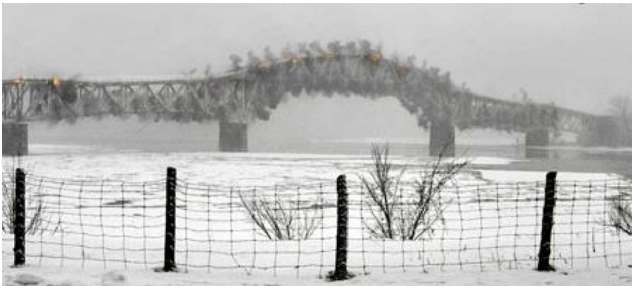
Demolition of the Lake Champlain Bridge, December 28, 2009
