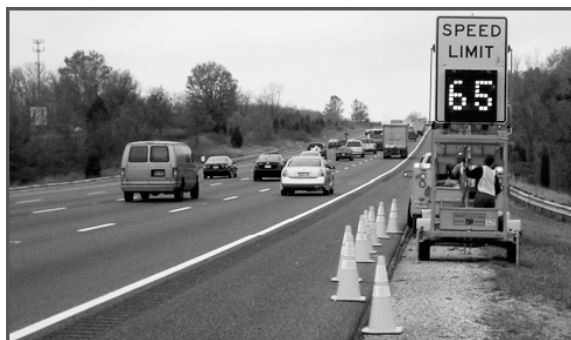
VSL trailer displays safe speed based on road work and traffic conditions
