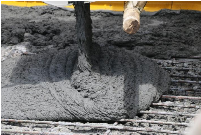
Figure 6. Photograph. Example of thixotropic UHPC mixture being placed for a UHPC overlay.
