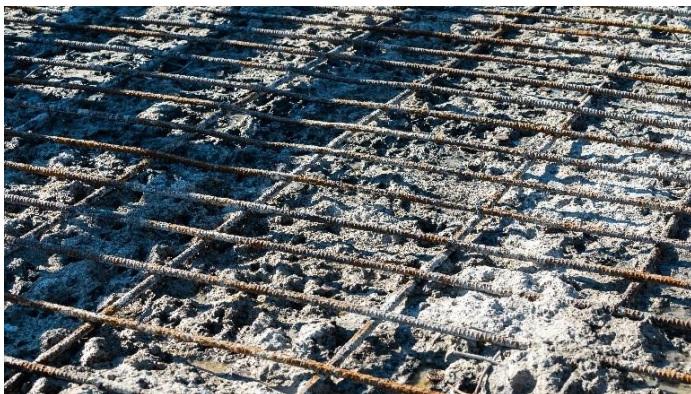
Figure 2. Photograph. Example of bridge deck after hydromilling process.
