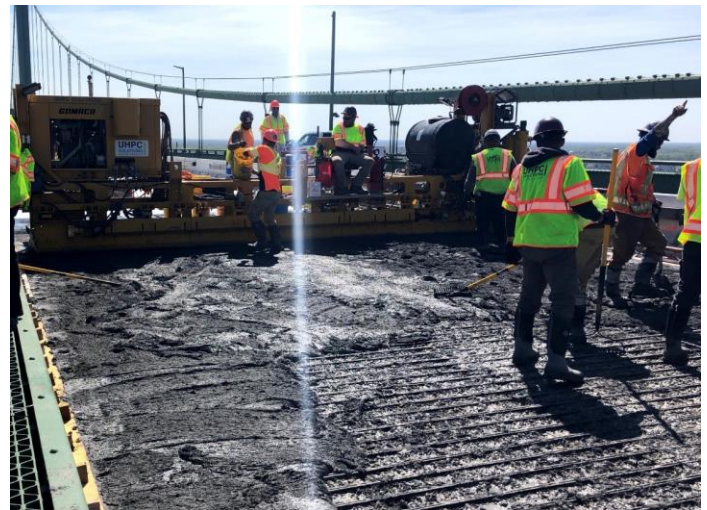
Figure 8. Photograph. UHPC overlay being placed with specialized paving equipment.
