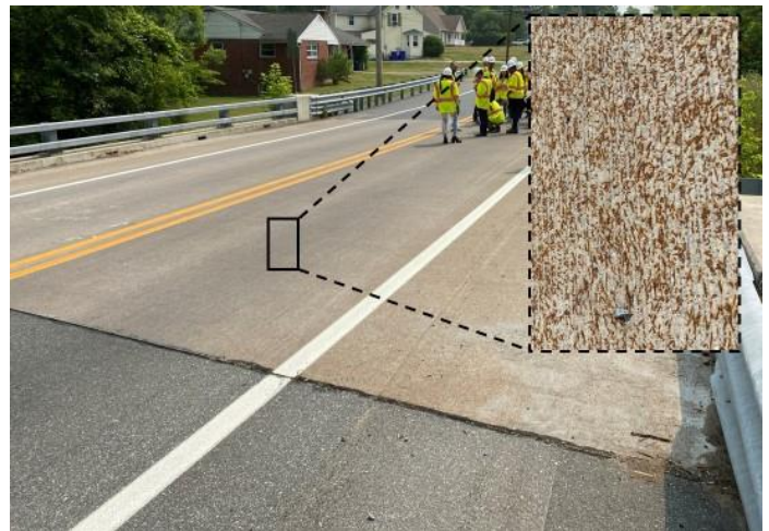
Figure 13. Photograph. Example of a finished riding surface after grinding and grooving.
