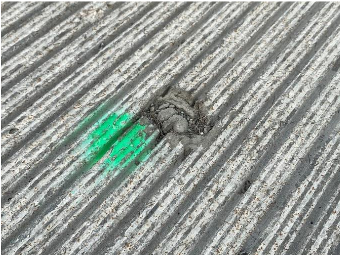
Figure 7. Photograph. Example of fiber ball in finished overlay after grooving.
