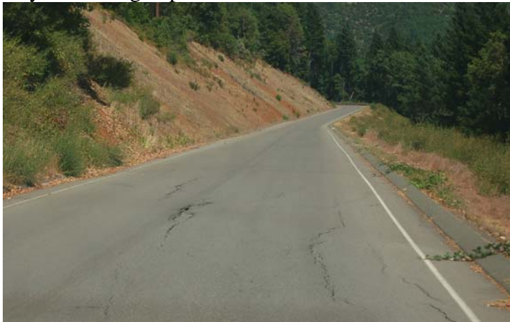
Pavement damage at slide area
