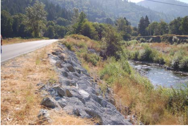
Newly constructed roadway and riprap along river
