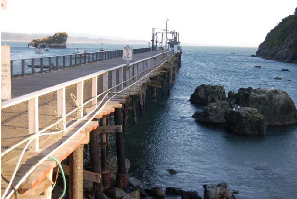
Pier at Trinidad Rancheria
