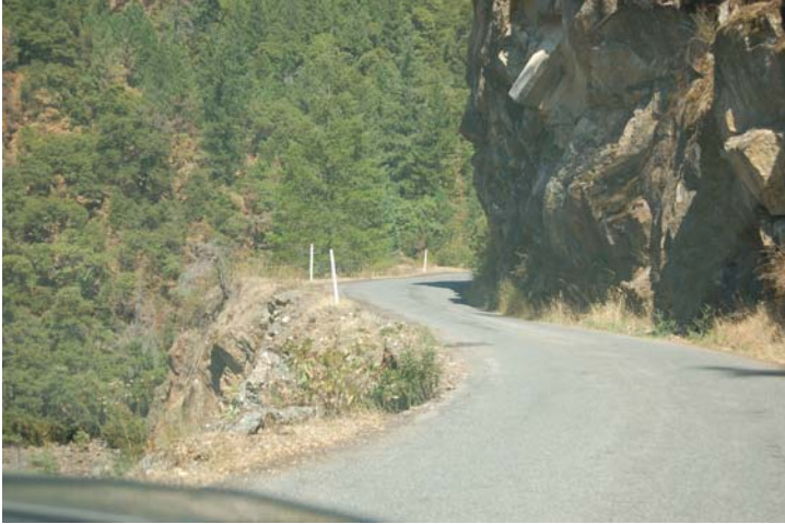
Salmon River Road – one lane road
