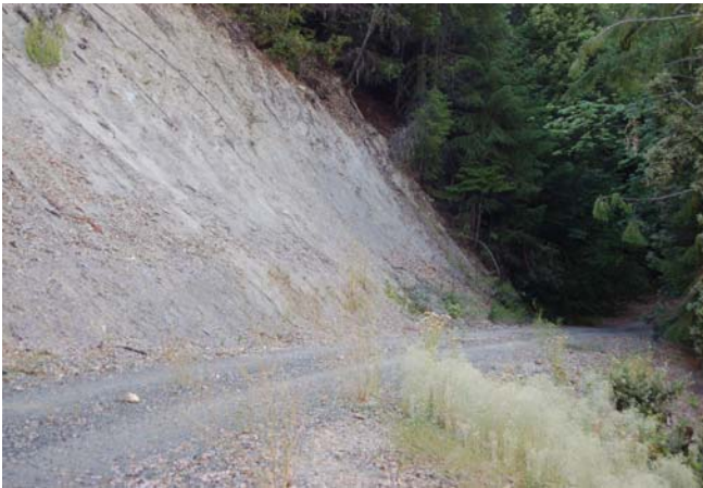
Multi-plate and roadway at newly constructed project
