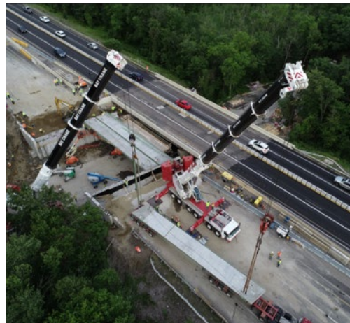
Figure 9. UAS monitoring of active construction projects. (Source: MassDOT)
