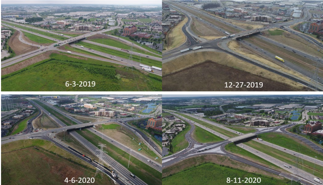
Figure 2. UAS-collected construction progress monitoring images.(Source: ODOT)
