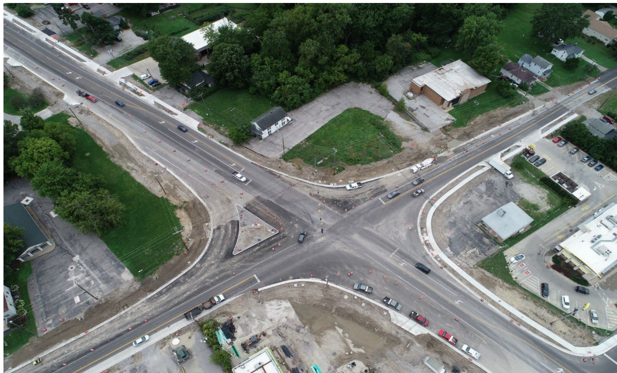
Figure 3. ODOT used UAS to assist with placement of traffic control equipment to increase safety.(Source: ODOT)
