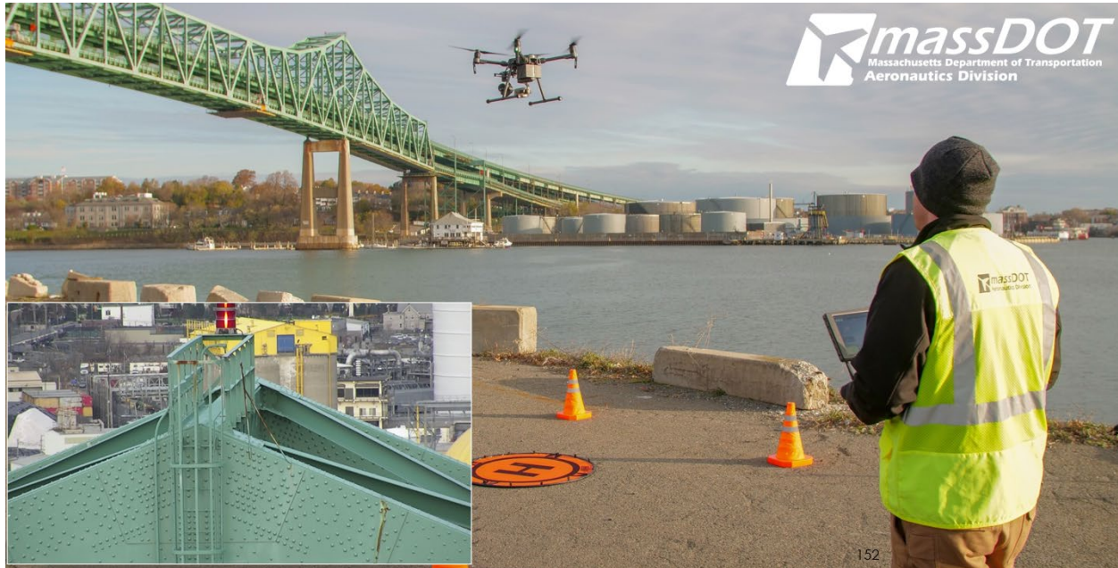
Figure 8. MassDOT use UAS on bridge inspections to reduce work zones. (Source: MassDOT)
