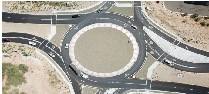
Figure 1. SR-60 Cherry Creek Roundabout UAS Data Collection (Image ADOT)
