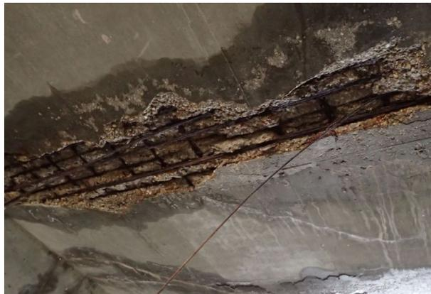
Figure 12. Deteriorating Culvert Infrastructure. (Source: NMDOT)
