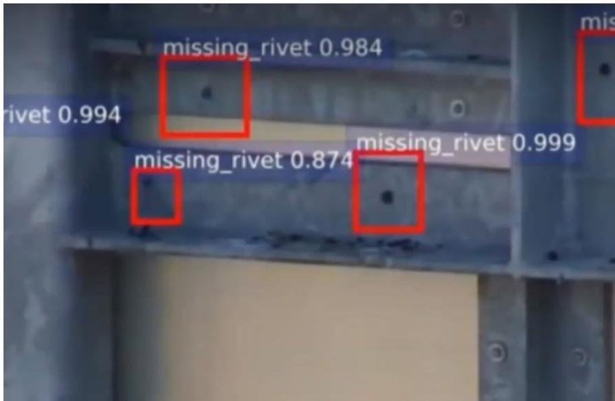
Figure 22. Machine Learning Detecting Missing Rivets on UAS Collected Data. (Source: UDOT)
