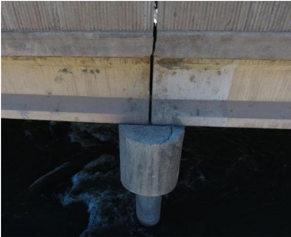
**Figure 18. Cracked Substructure Support on Large Bridge. (Source: UDOT)**
