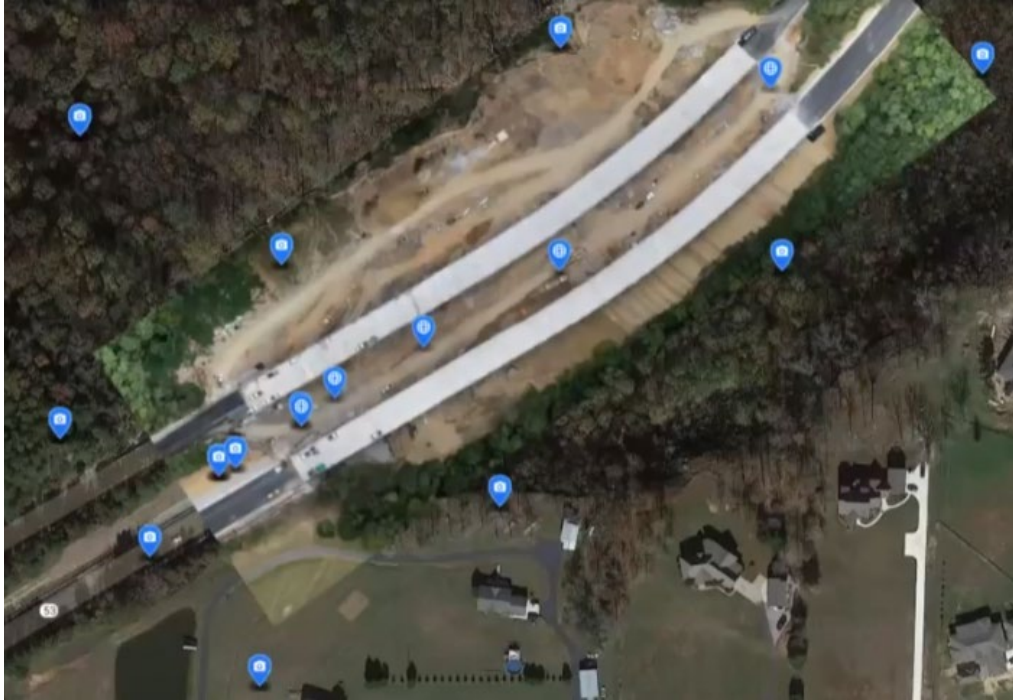
Figure 5. UAS Software Project Progress Report with Links (Source: Alabama DOT)
