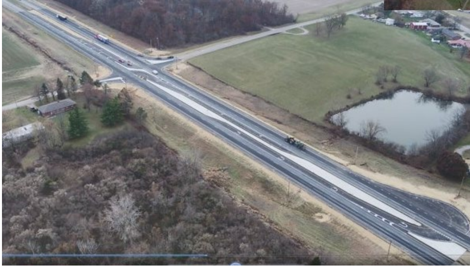
Figure 8. UAS Image of a New Roadway Design Project (Source: Ohio DOT)
