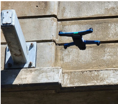
Figure 10. MnDOT Demonstrating Various UAS Platforms for Bridge Inspections. (Source: FHWA)
