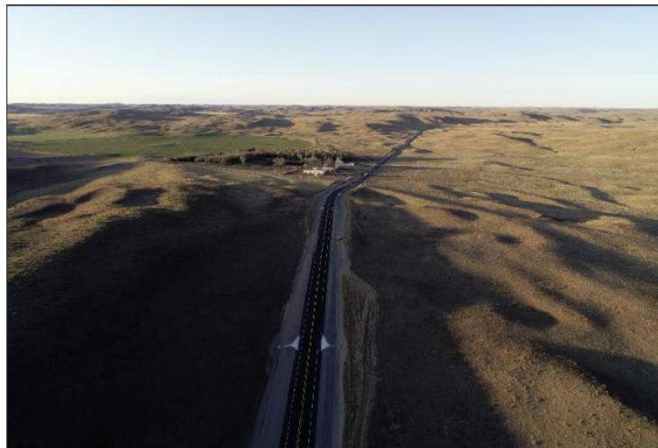
Figure 4. NDOT UAS Footage. (Source: NDOT)
