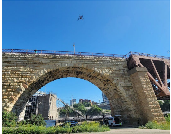
Figure 9. MnDOT UAS Bridge Inspection Demonstration. (Source: FHWA)
