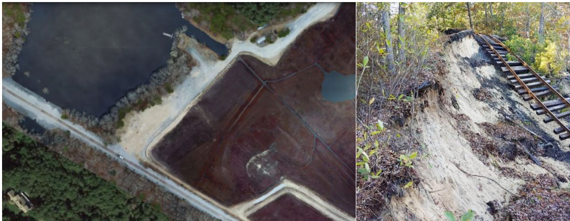
Figure 3. Cranberry Bogs Compromised Railway. (Source: MassDOT)
