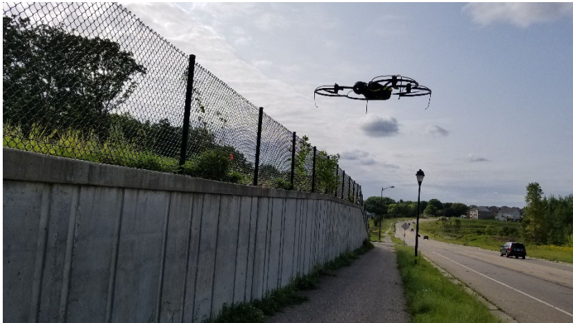
Figure 1. MnDOT Retaining Wall Inspection Using UAS (Photo Courtesy MnDOT)
