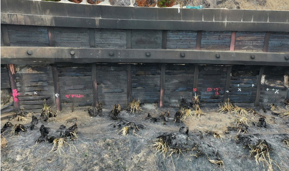
Figure 7. 3D model of post fire response north of Jenner, California (Photo courtesy of Caltrans Steep Terrain UAS Group)
