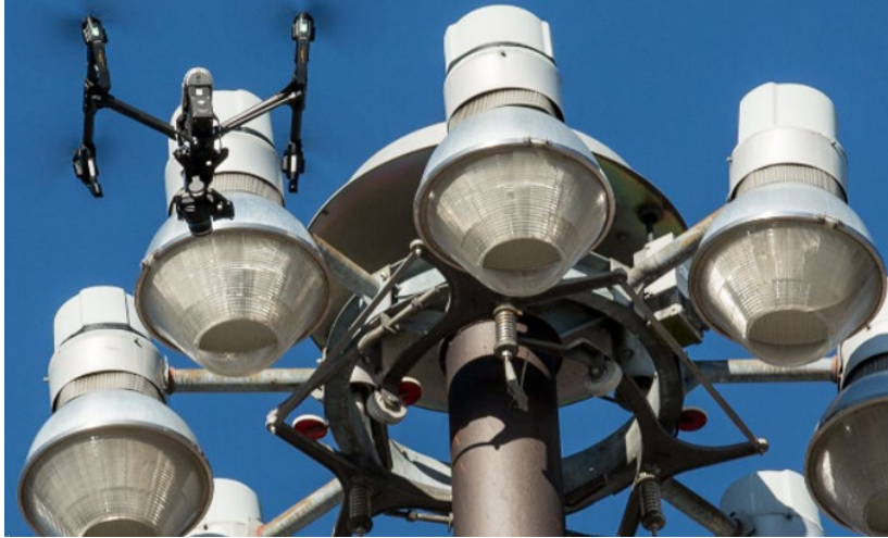
Figure 1. UAS Inspecting HMLP. Source: NJDOT
