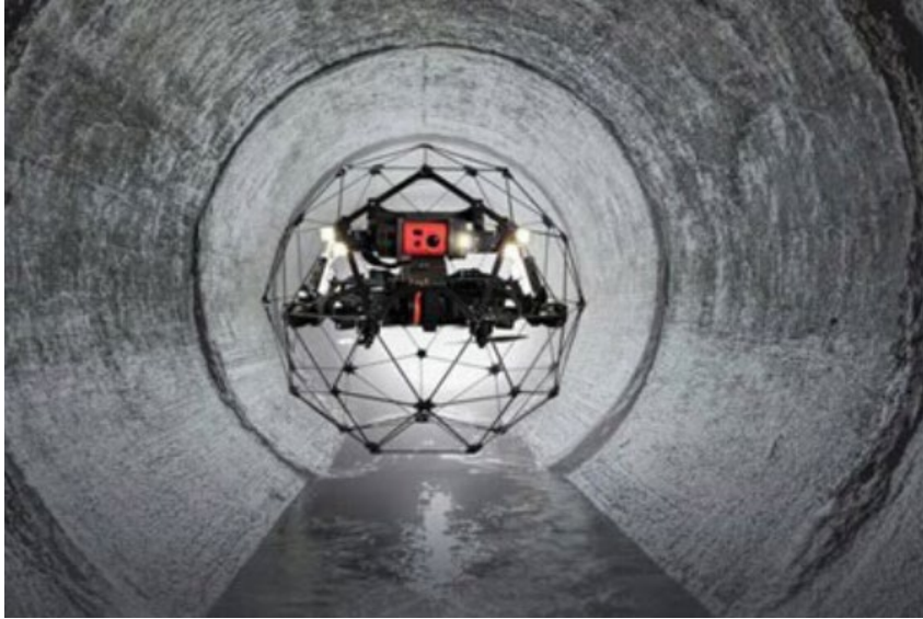
Figure 5. UAS Inspection of Large Pipe. Source: MDOT
