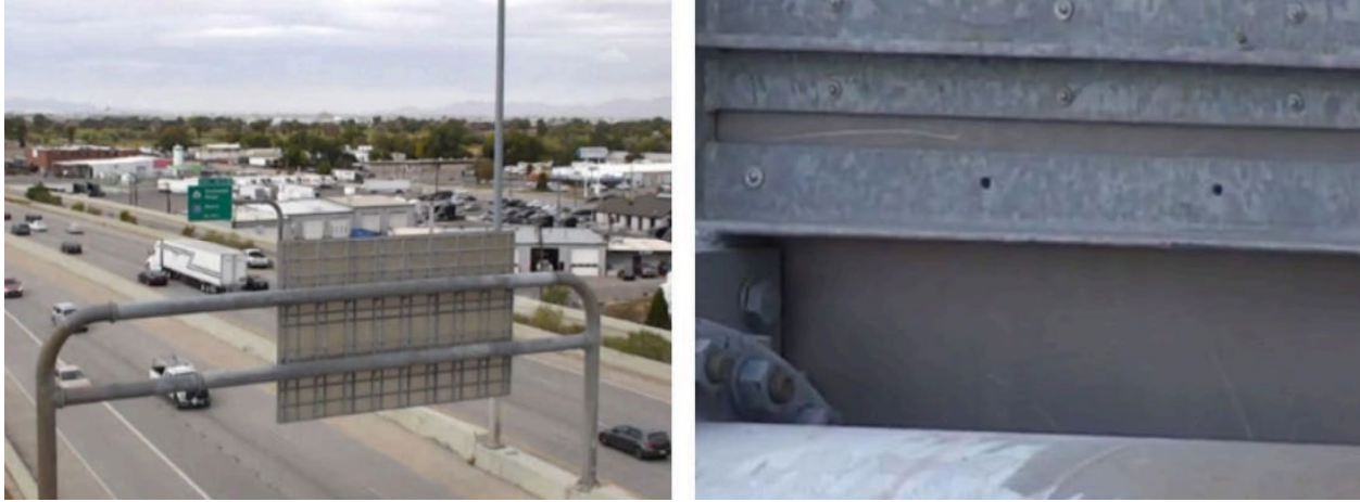
Figure 6. UAS Overhead Sign Inspection. Source: UDOT
