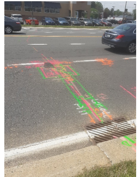
Designating underground utilities. Photo: DelDOT
