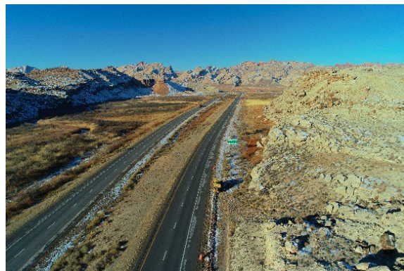
A trench for fiber conduit along I-84 in Utah. Photo: UDOT
