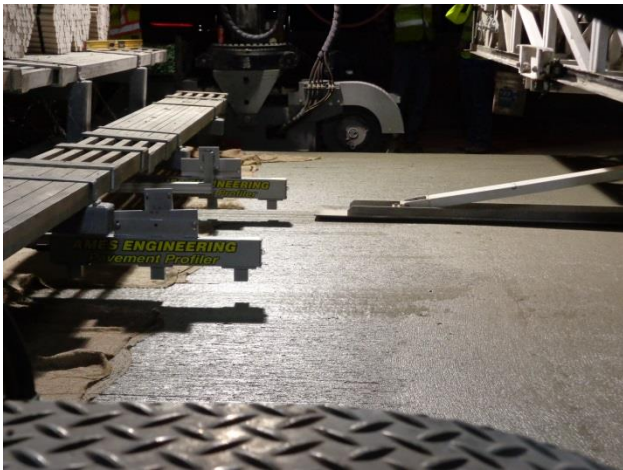
Figure 1. Ames RTP Mounted to G-Z S-850 Paver With a Float Pan
