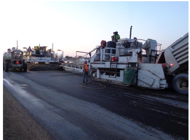
Figure 2. Trucks Dumping Concrete at Gomaco 9500 Placer, Installation of Dowel Baskets and Concrete Deposited Ahead of the Paver
