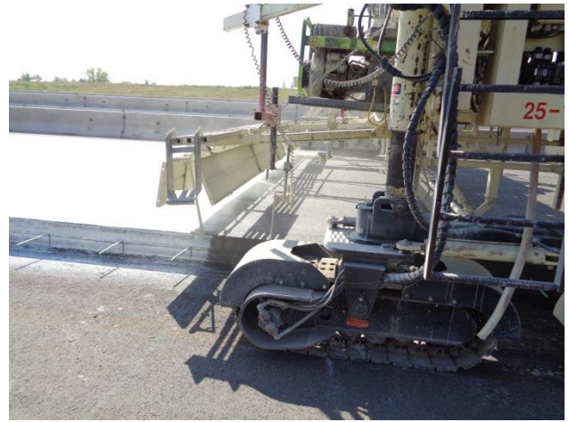
Figure 6. Application of Curing Compound
